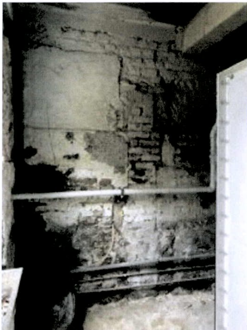
Plate 100: Former kitchen to northwest at basement level, with original masonry and floor flags evident. Note concrete downstand beam for concrete floor plate supporting entrance level above
