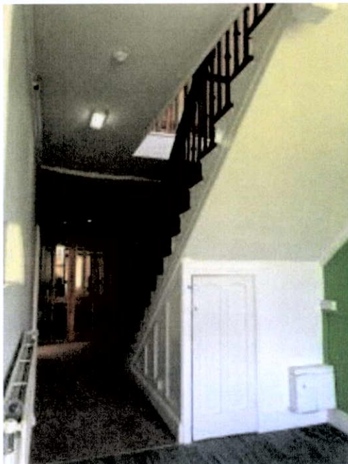
Plate 209: Open tread, timber stair in north-east bay. Turned newel post and timber handrail.
