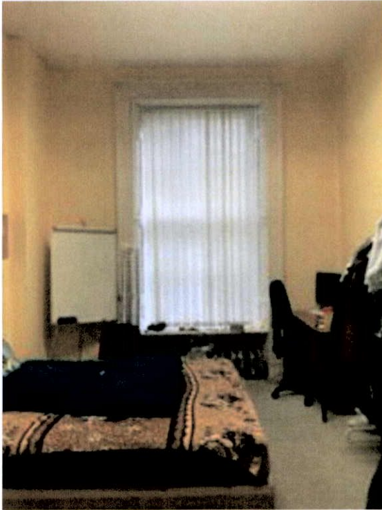
Plate 114: Typical cellular room on the upper level. Panelled door, sash window with moulded architrave. No decorative plasterwork.
