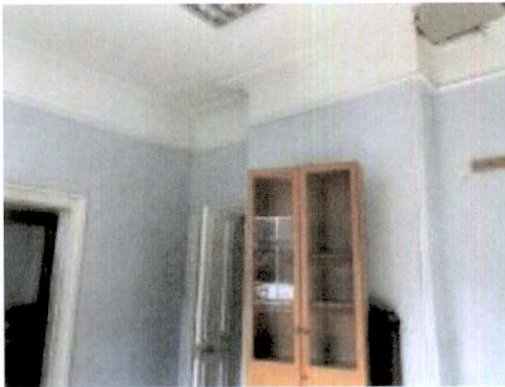
Plate 197: Stepped cornice and picture rail in ground floor accommodation.
