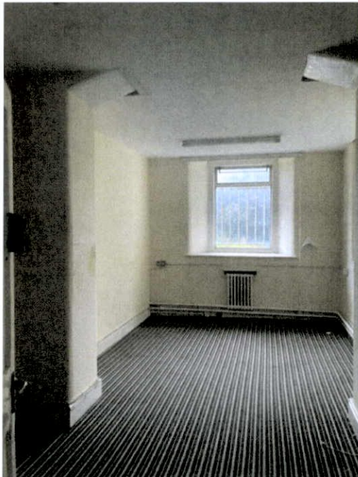
Plate 303: Lowered ceiling. Arched openings supporting columns in Chapel above. Contemporary windows. No decorative plasterwork.
