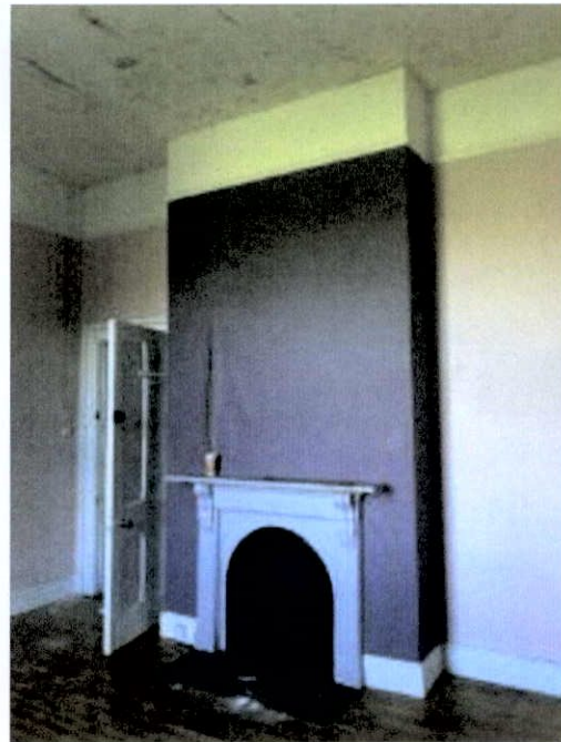
Plate 194: Corbel chimneypiece and cast iron insert. Paneled door, molded architrave and picture rail.
