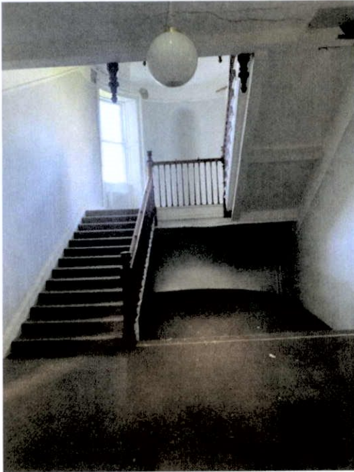
Plate 281: Main stairs with open well within rounded bay to rear (north) of Tabor House
