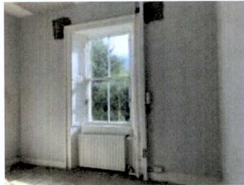
Plate 198: Two-over-two sash window, original shutters and architrave. Areas of plaster removed to reveal underlying masonry substrate.
