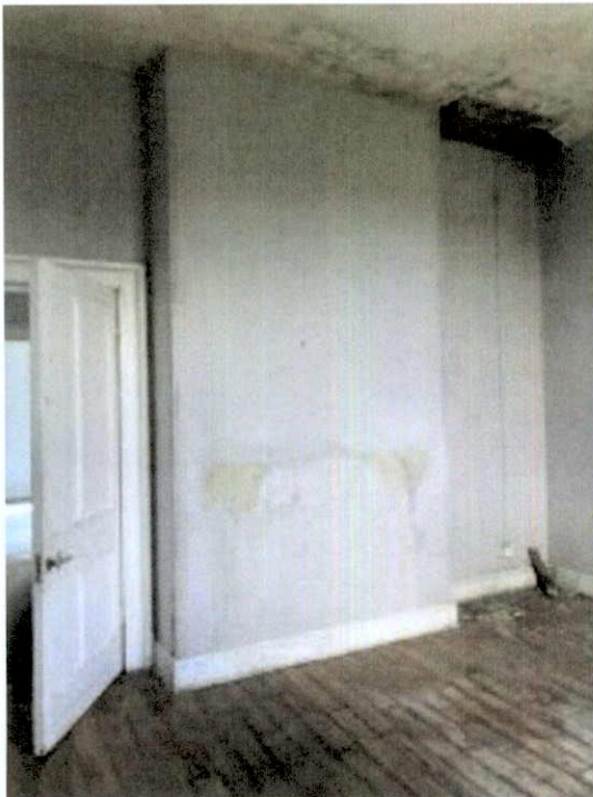
Plate 253: Chimneybreast with chimney piece removed. Evidence of water damage to ceilings and walls.
