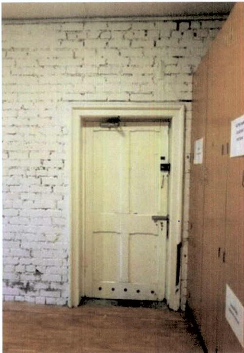
Plate 229: Services area at lower ground floor level with original walls exposed and painted. Original panelled door.
