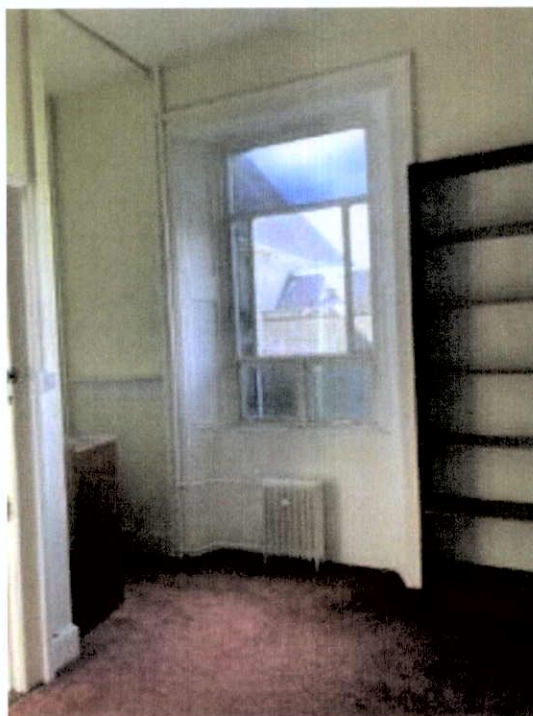
Plate 253: Chimneybreast with chimney piece removed. Evidence of water damage to ceilings and walls.
