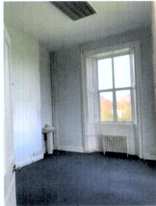
Plate 248: Typical first floor accommodation, original window-box with contemporary uPVC window. Exposed services, no decorative plasterwork.
