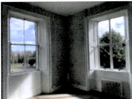
Plate 251: Dormitory with original window-box and two-over-two timber sash.
