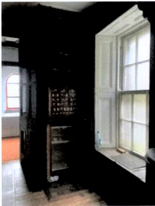
Plate 316: Six-over-six timber sash within sacristy.
