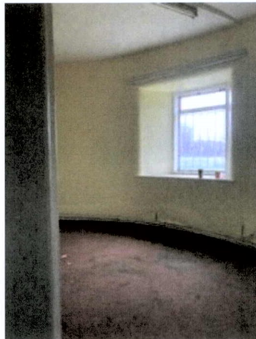
Plate 312: Lower ground floor, within rounded bay. Evidence of water ingress at base of walls.
