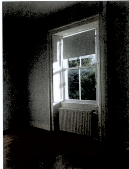
Plate 250: Dormitory with laminate flooring. Original window-box and two-over-two timber sash.
