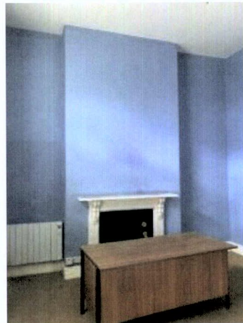
Plate 200: Corbel chimneypiece and cast iron insert. No cornice.
