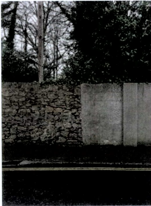
Plate 78: Change in wall composition on Milltown Road near junction with Sandford Road. Rubble wall is rendered and meets later pier
