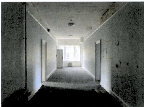
Plate 275: Central spine corridor. Original timber floor under carpet finish. Staining to ceiling evident.
