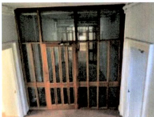
Plate 205: Entrance level corridor with later cross-corridor fire screens. Water ingress damage to ceiling fabric.
