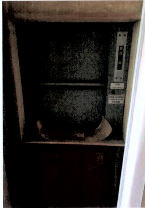
Plate 230: Dumb waiter from kitchen to dining area
