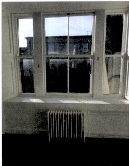
Plate 263: Detail of tripartite sash window.
