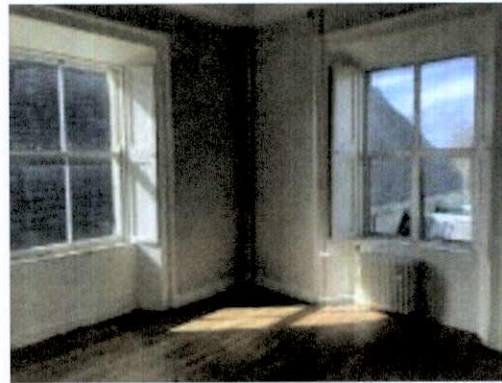
Plate 278: Original window joinery, with contemporary uPVC window frame in north elevation.
