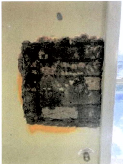
Plate 123: Opening up investigations to uncover brick substrate.
