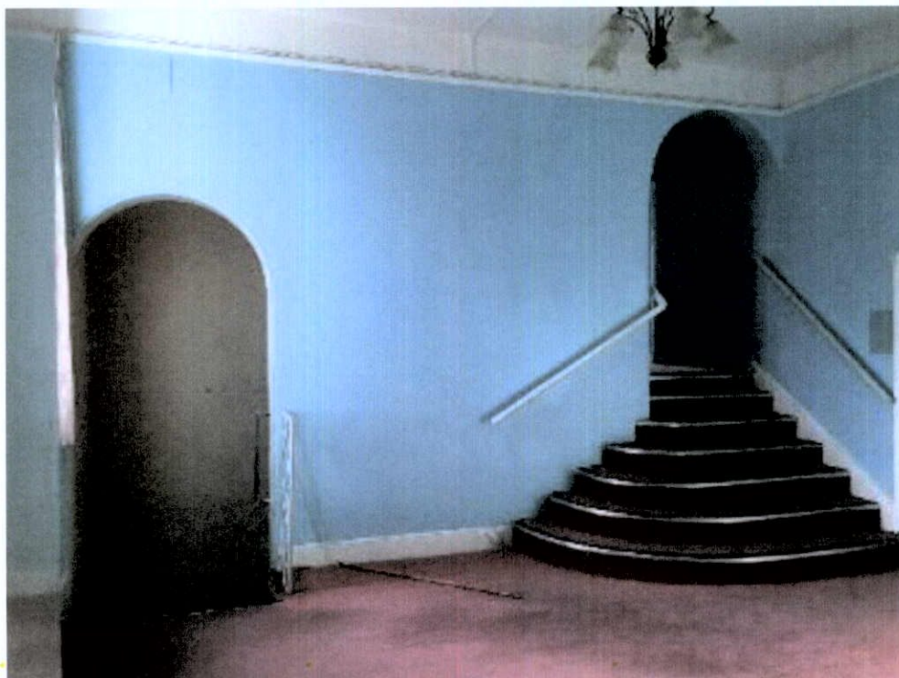
Plate 105: First floor level infilled entrance hall with later stairs leading to vertical extension.
