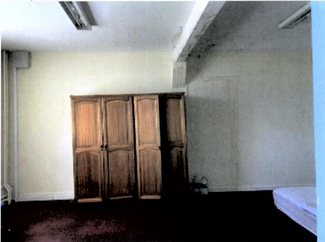
Plate 116: Amalgamated room, with beam supporting structure on level over. Evidence of water ingress. Exposed services. No chimneypiece or historic plasterwork.
