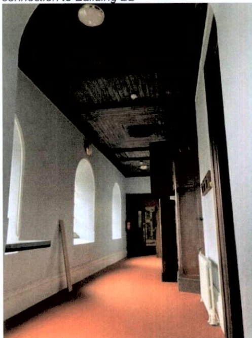
Plate 309: Detail of timber panelled ceiling.
