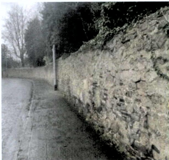
Plate 80: Curve of wall looking up Milltown Road towards new entrance, note multiple pointing types cement repairs to rubble wall
