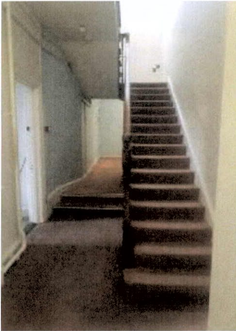
Plate 173: Stair at rear of block. Timber, open tread with turned bannisters.
