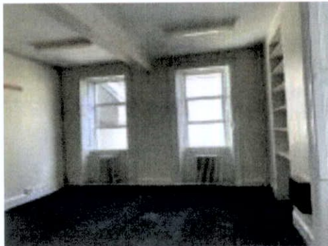
Plate 144: Later windows with original panelled shutters, exposed grid structure.
