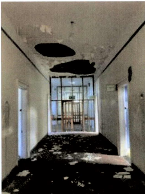
Plate 205: Entrance level corridor with later cross-corridor fire screens. Water ingress damage to ceiling fabric.
