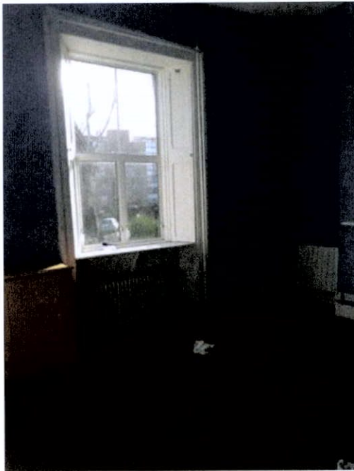
Plate 249: Dormitory facing south east, original window-box with contemporary uPVC window.
