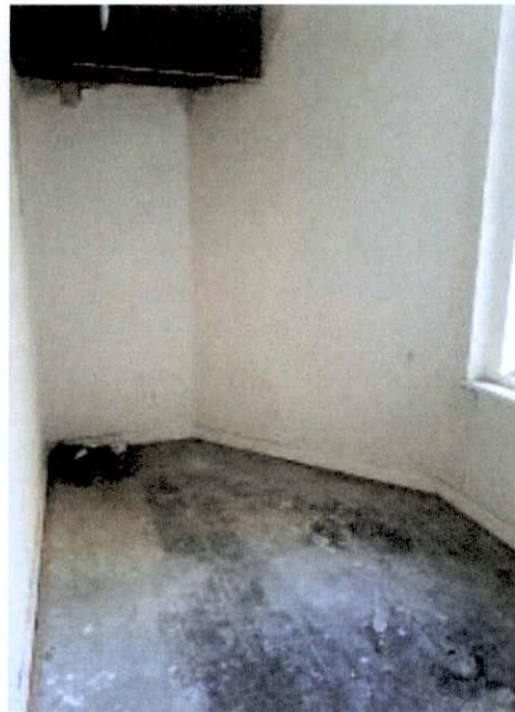
Plate 141: Small room with partitioned wall showing signs of water damage
