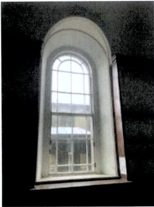
Plate 156: Round headed timber sash window with margin lights within former domestic Chapel.
