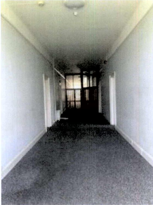
Plate 245: Central corridor with later fire-rated screens across corridors and enclosing stairs.
