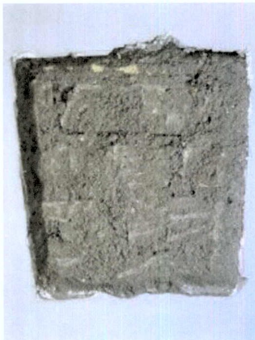
Plate 199: Section of plaster removed to reveal brick substrate.
