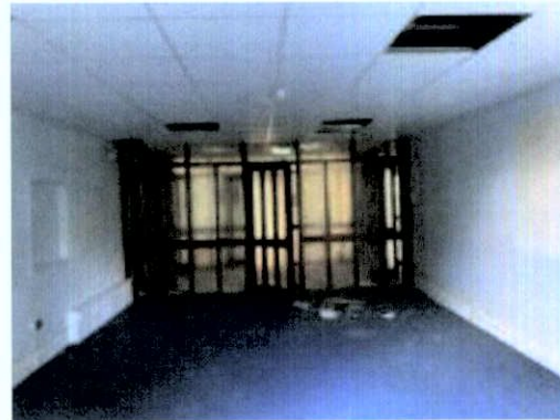
Plate 238: Later timber-framed fire screens within corridor.
