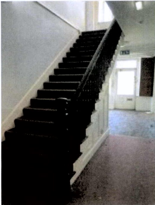
Plate 209: Open tread, timber stair in north-east bay. Turned newel post and timber handrail.
