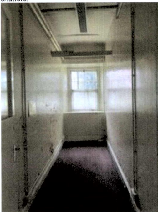
Plate 305: Lower ground floor corridor with exposed services. Original sash windows and shutters.
