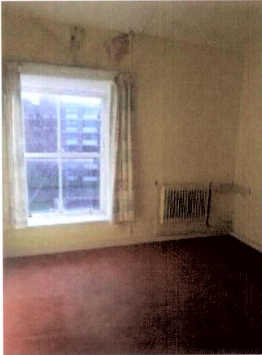
Plate 177: 2 nd floor level typical study room to front (east) on first floor with signs of water damage
